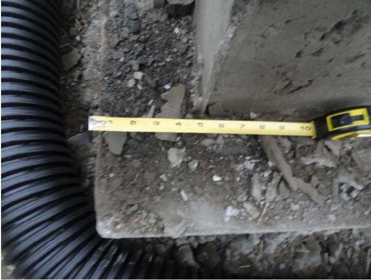
Footings projection SE corner
