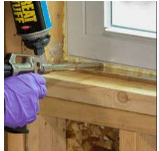
Spray foam being installed in the rough opening gap
