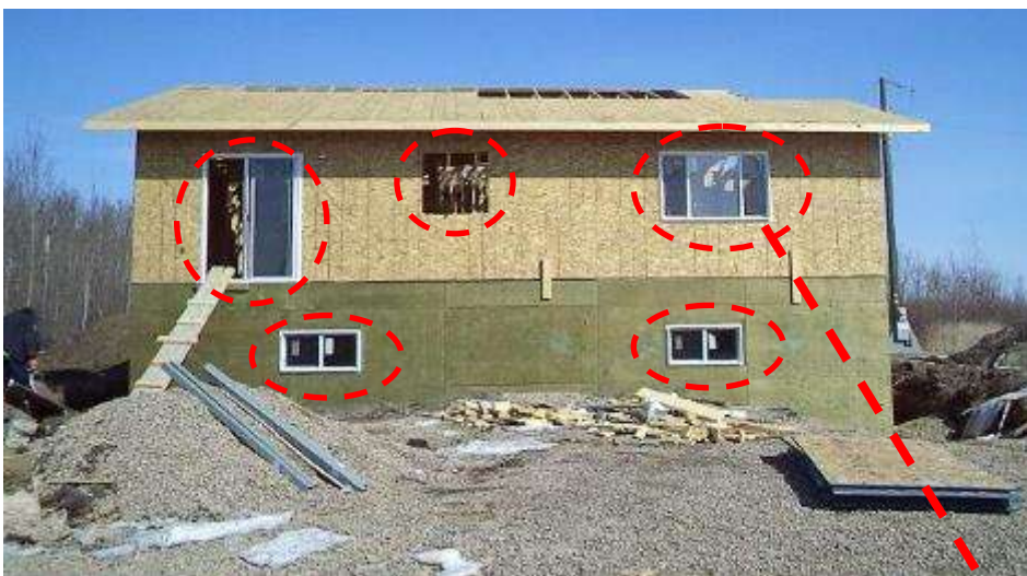
Windows installed directly into a bare wood-framed wall
