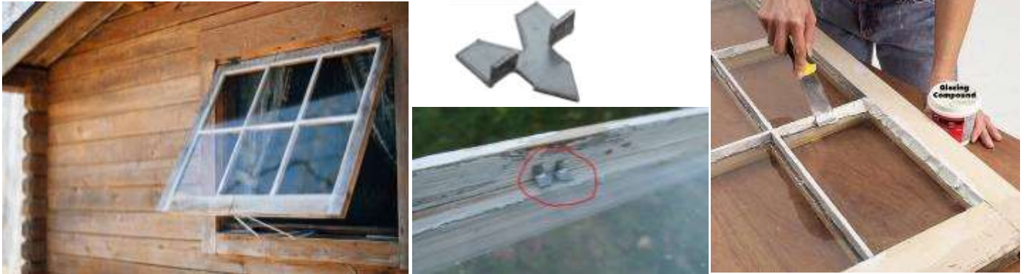
An old traditional-style, wood-framed window with multiple small single panes of glass held in place with wood muntins, steel glazing points, and glazing putty
