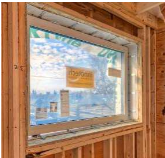
Window with strap anchors built into the frame installed in a rough opening
