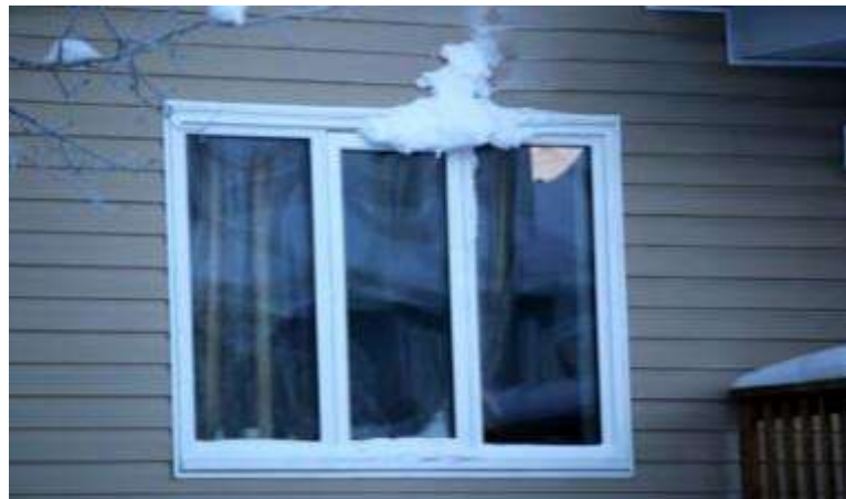
Ice formation from air leakage at the window header
