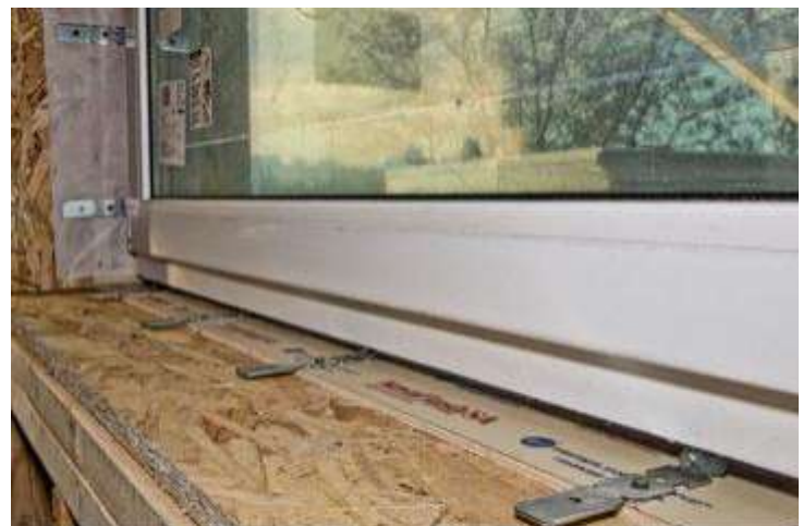
Window with strap anchors built into the frame installed in a rough opening
