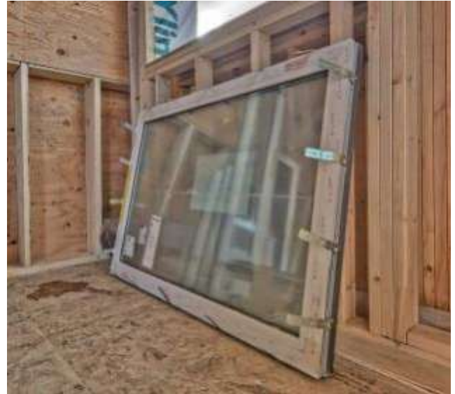
Window with strap anchors built into the frame
