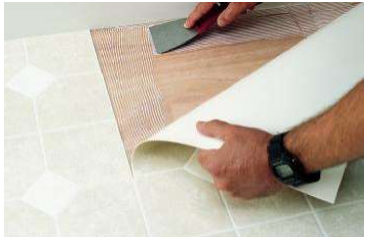
Vinyl-sheet flooring being installed
