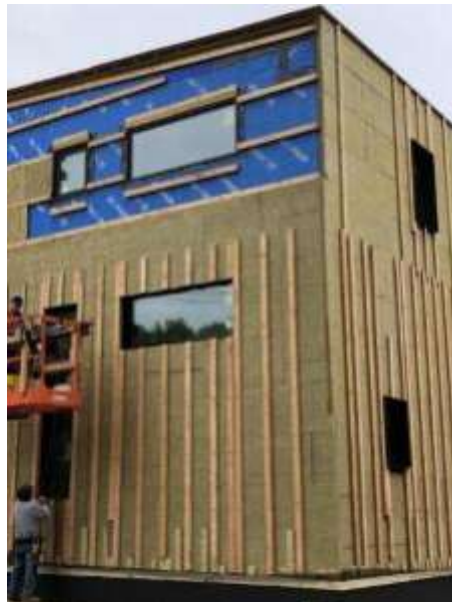
Board mineral fibre installed on the exterior of a wall
