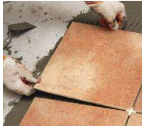
Ceramic tile being installed
