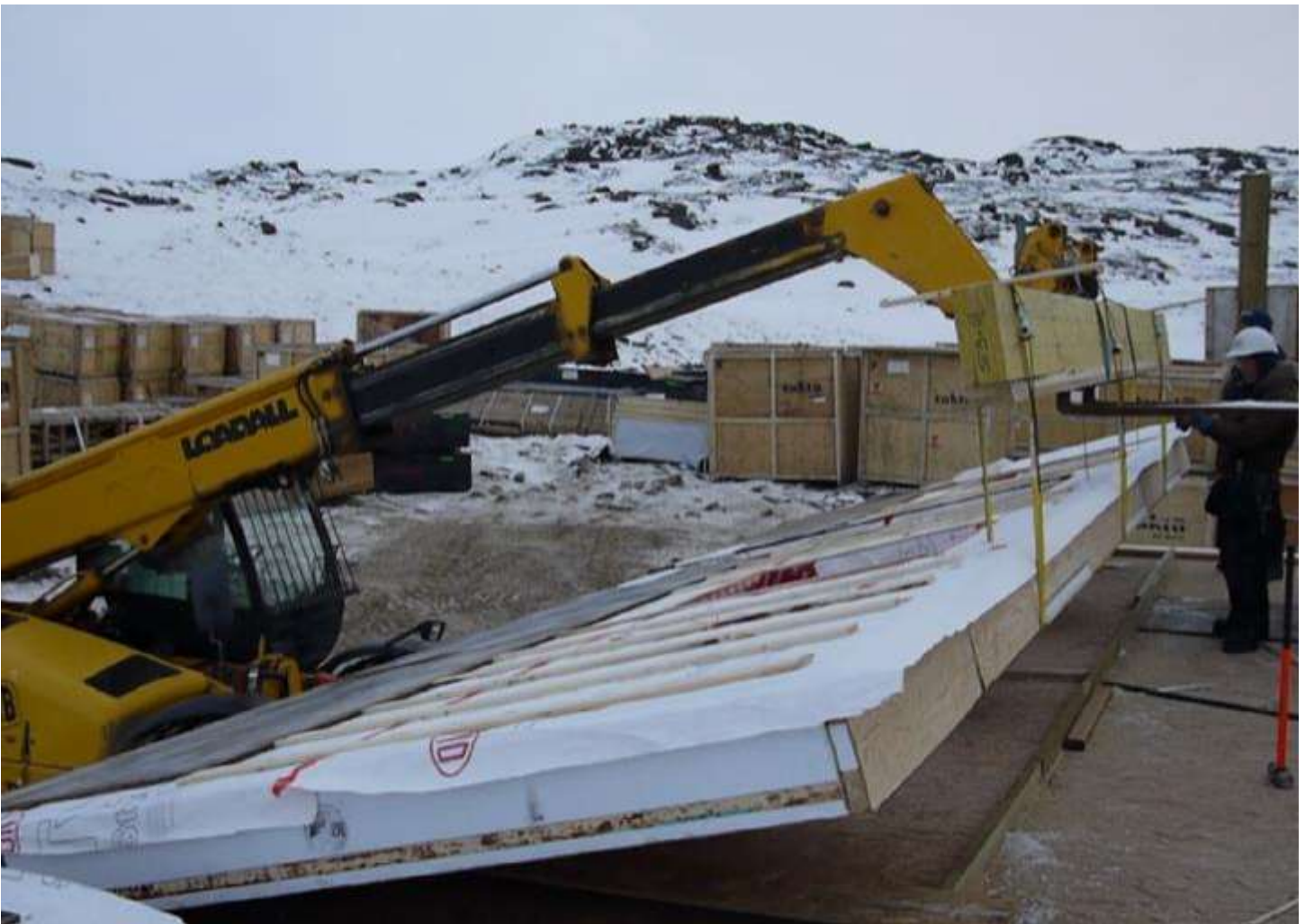
A premanufactured panel wall being lifted into place
