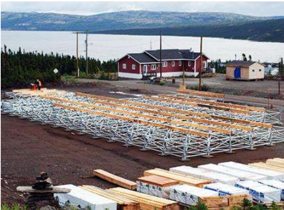
Wood-floor framing being constructed on a space frame foundation
