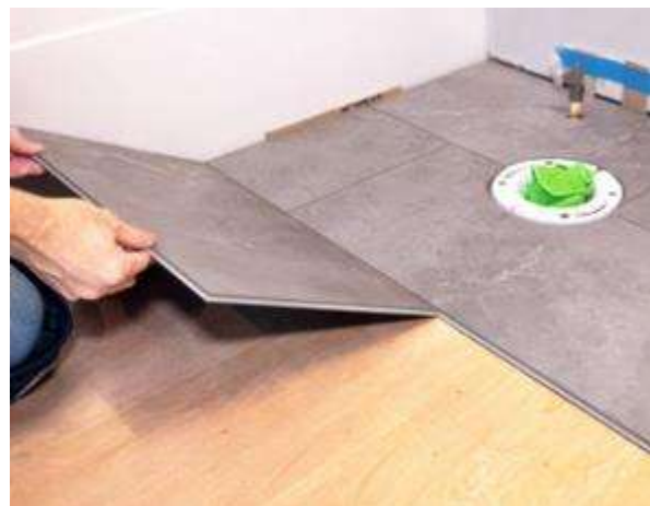
Vinyl-tile flooring being installed
