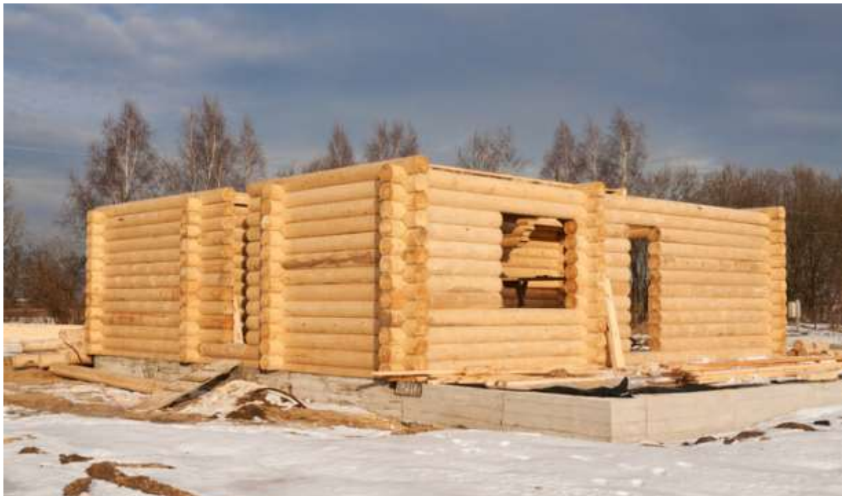
A log house under construction
