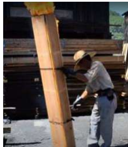
Wood siding being charred
