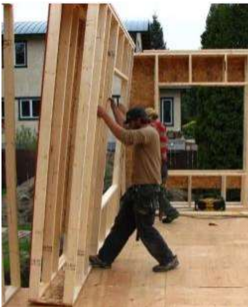
Double-stud wall being tilted into place
