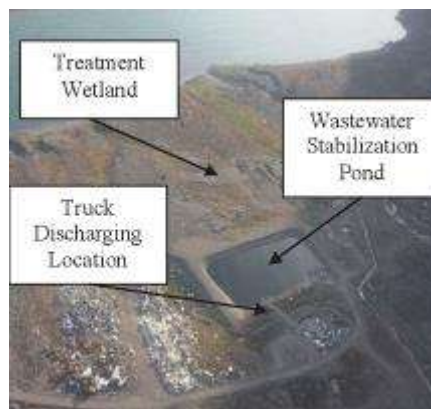
A sewage lagoon with a single pond that flows into a wetland
