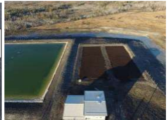
A sewage lagoon with multiple ponds
