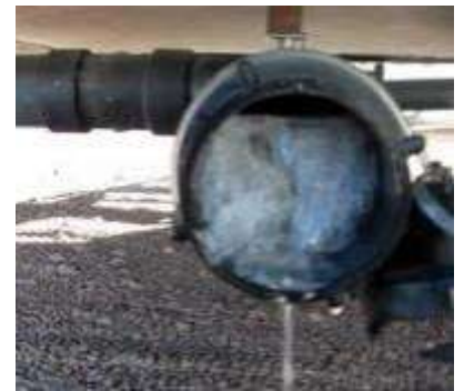
A frozen pipe filled with ice
