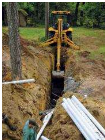
Septic pipe trench between the tank and field
