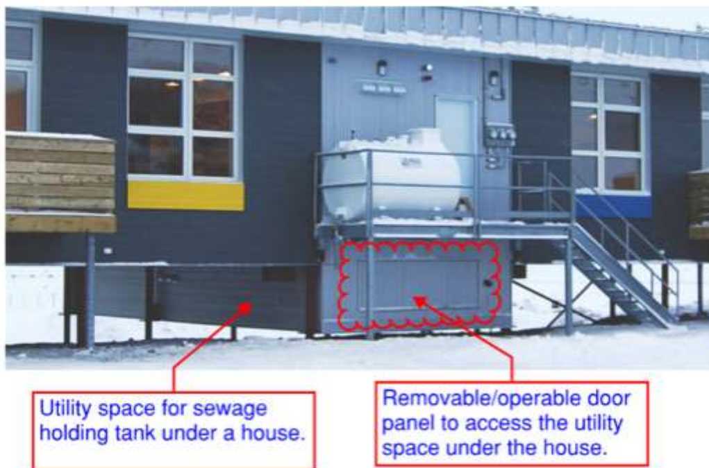
A utility space under a house with a removable/operable door panel
