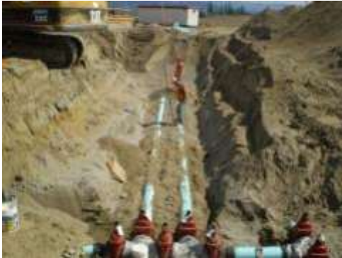
Water supply pipes being installed in a trench
