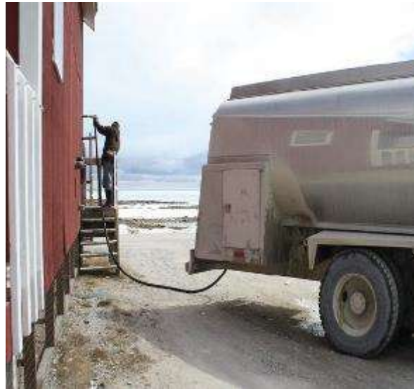
Worker filling up a house's water tank at the fill port with a hose from the water delivery truck
