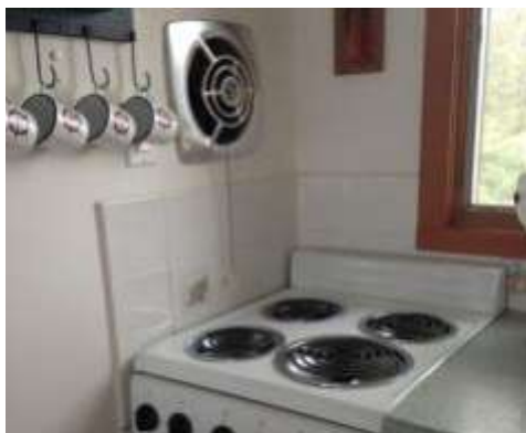
A basic exhaust fan over a stove
