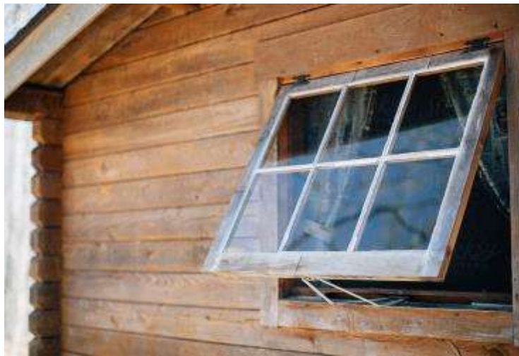
Natural ventilation through an open window
