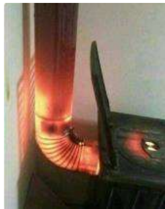
Burning creosote deposits in a chimney causing the chimney to overheat and glow red hot
