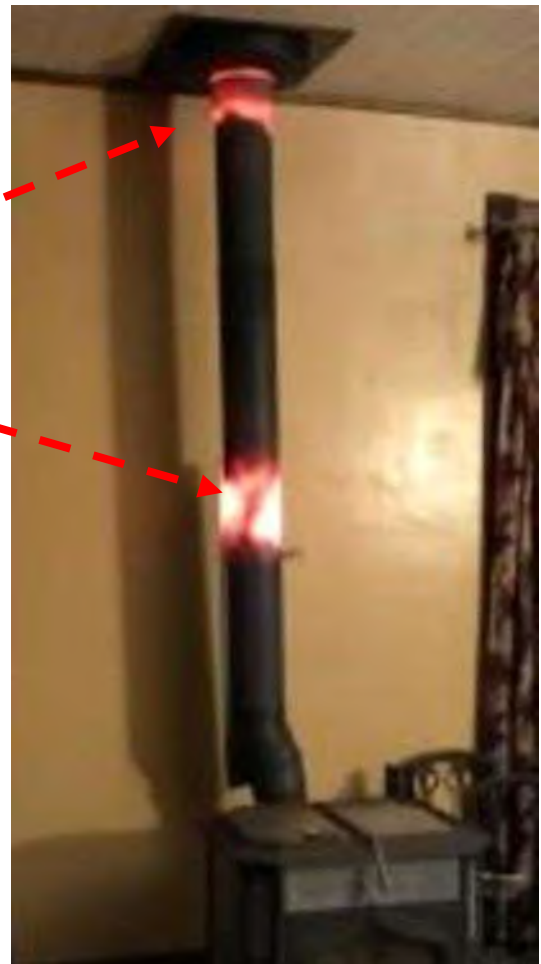
Burning creosote deposits in a chimney causing the chimney to overheat and glow red hot
