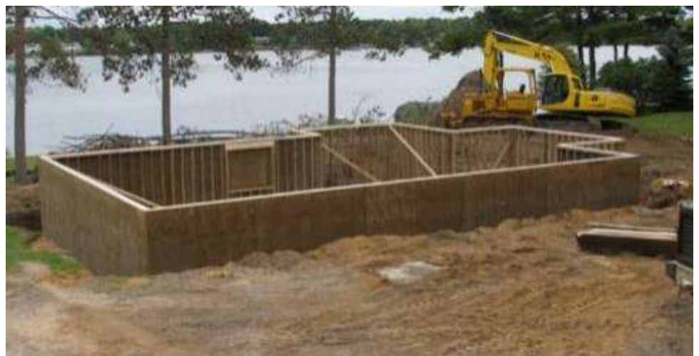
A basement constructed with wood framing
