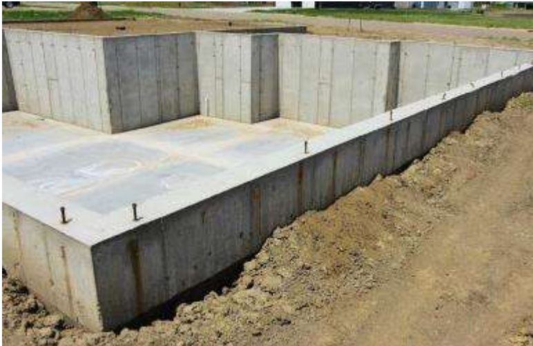
Typical basement constructed with cast-in-place concrete
