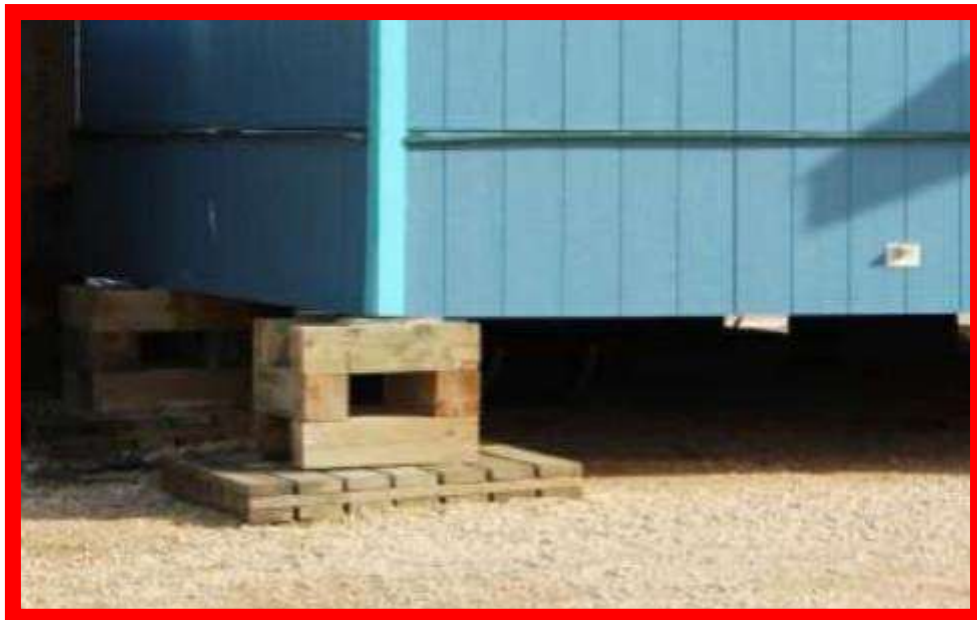
A house with a wood cribbing foundation
