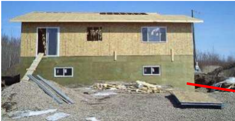
House being constructed with a wood-framed basement
