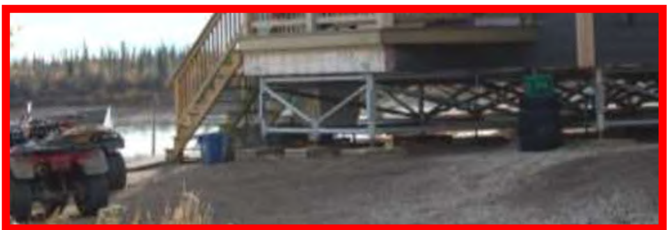
House with a steel space-frame foundation
