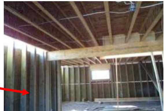
Interior view of wood-framed basement under construction
