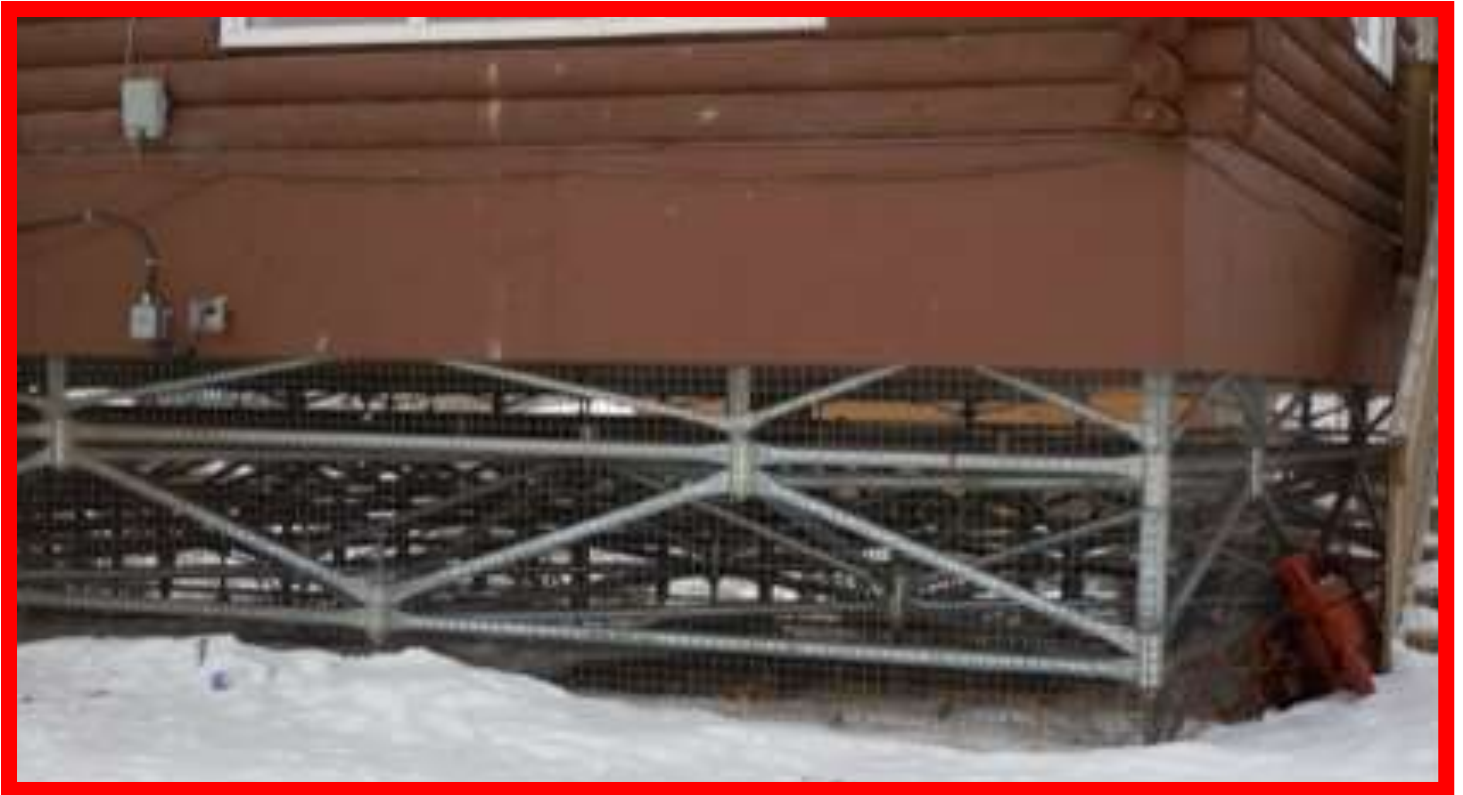
House with a steel space-frame foundation
